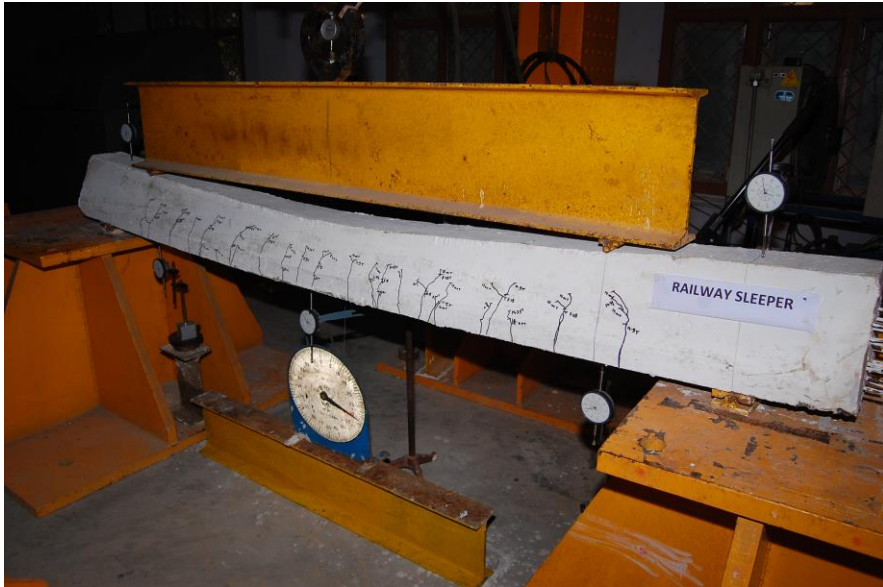
Fig. 32 Crack Pattern of GPC Sleeper
