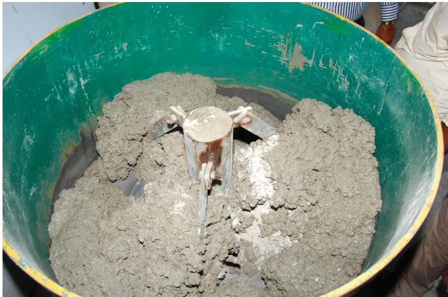
Fig. 6 Mixing of Geopolymer Concrete
