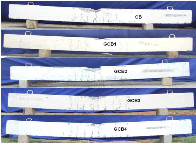
Fig.22 Crack Pattern of Beams
