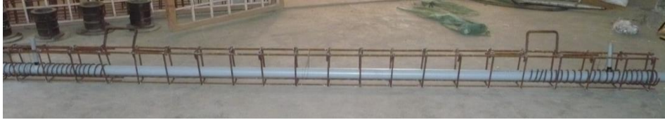
Fig. 33 Arrangement of Duct Before Casting
