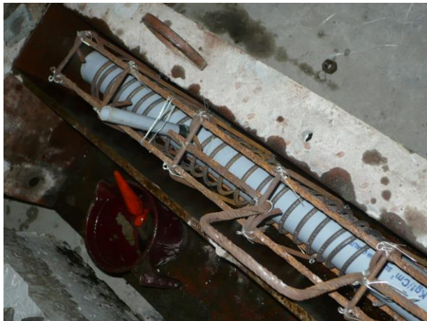
Fig. 34 Casting of Post Tensioned Beam
