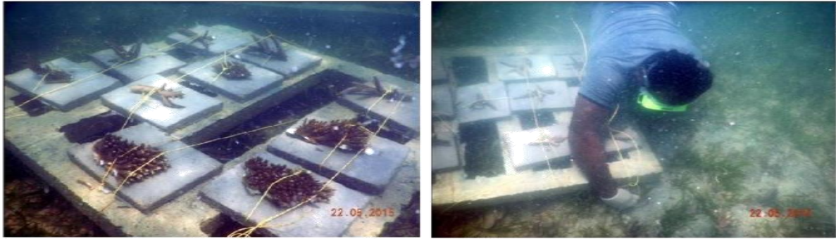
Placing of slabs with fixed coral fragments on the concrete frames
