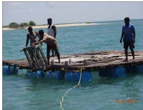
Transportation and deployment of substrates using raft
