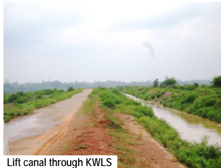
Lift canal through KWLS
