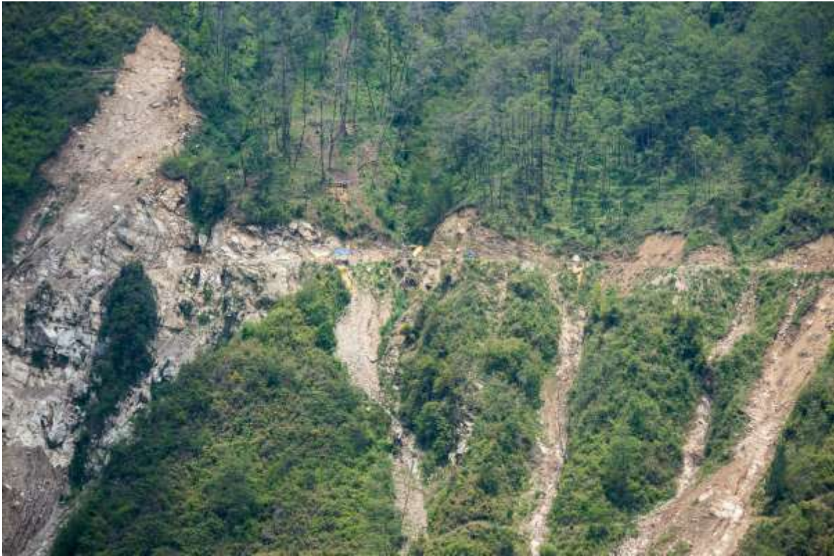
One of the roads and landslides that team has witnessed during the site inspection in Sikkim.
