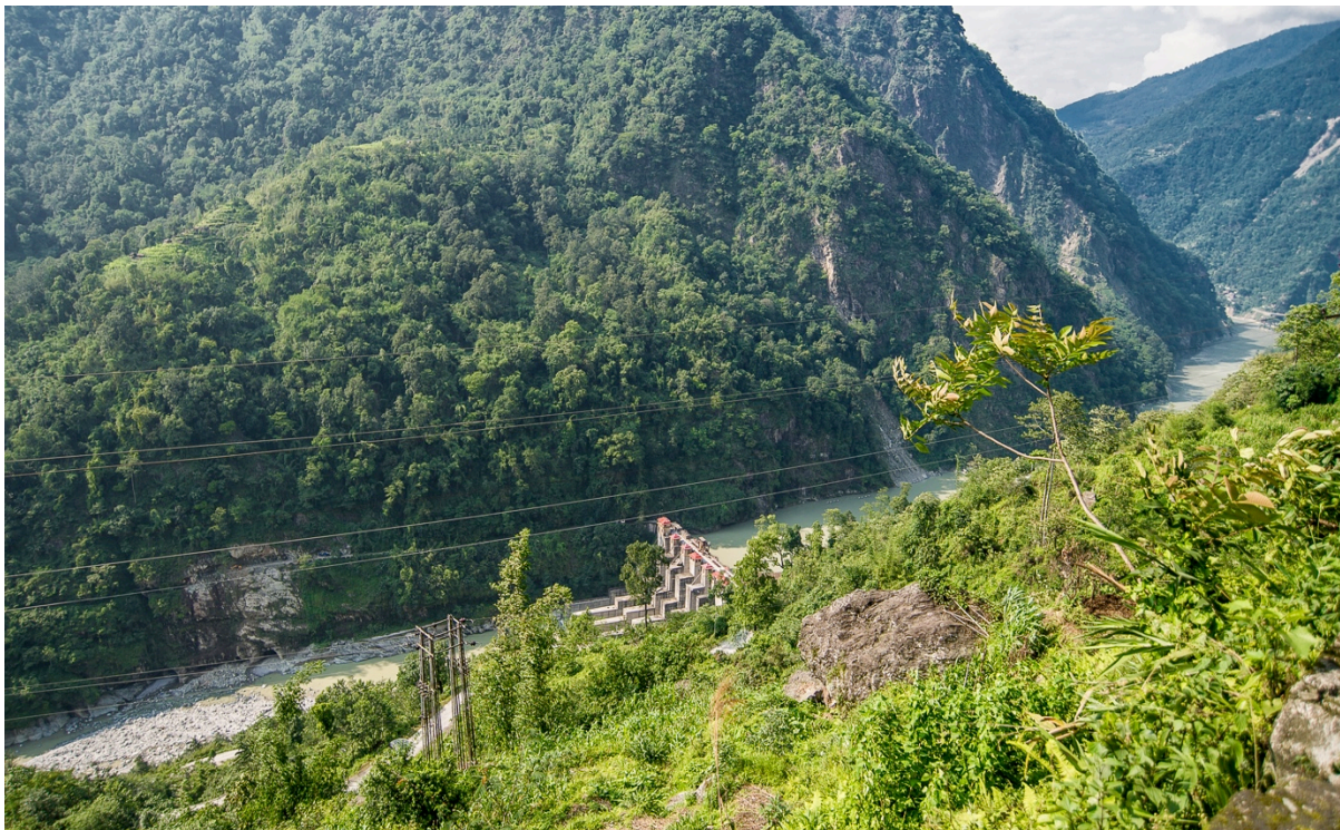
Figure 1: The Teesta V dam showing the virtual absence of flow in the river downstream of the dam, which can have devastating consequences for river-dwelling and river-dependent species.
