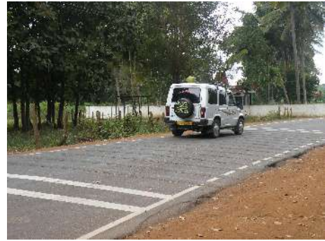
Speed breakers, humps, rumble strips deployed at intervals and crucial locations can check speeding and avert many roadkills (Photo: A. J. T. Johnsingh)
