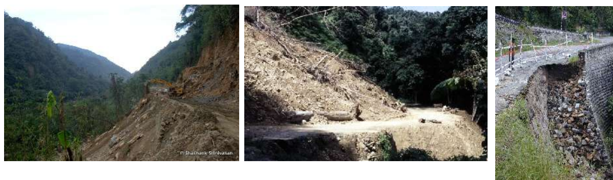
From left to right: Widening and earth dumping on road to Tawang near Pakke Tiger Reserve (Photo: Shashank Srinivasan); landslide on E-W Road in Great Nicobars (Photo: Manish Chandi); hard engineering methods are poor replacement for natural vegetation to prevent erosion and slips (Photo: NCF)
