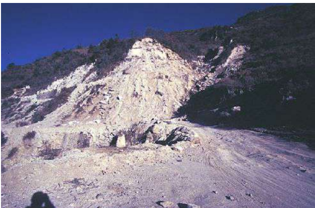
Huge landslides extending many hundreds of metres, in both forested and deforested slopes. Roads are cut with little thought to slope stabilisation. Given the very loose soil even the presence of trees does not always guarantee soil stability. Above: slides along a small track in Eaglenest sanctuary. Below: slides along the highway in Dirang and Jang.
