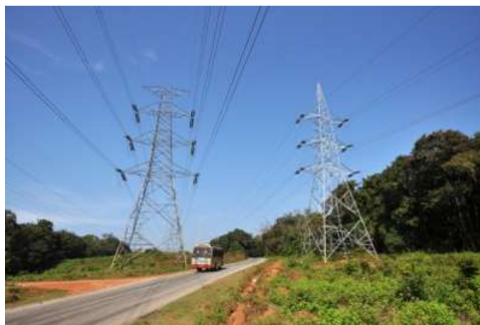
Transmission lines double up with a road through forests in Karnataka (Photo: NCF)
