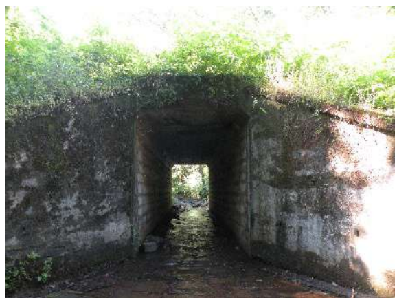
Effectiveness of existing underpasses such as this one below Dudhsagar railway track should be evaluated (Photo: A. J. T. Johnsingh)
