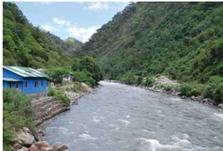
Figure II. 2.17: Near powerhouse site of Tawang-I
