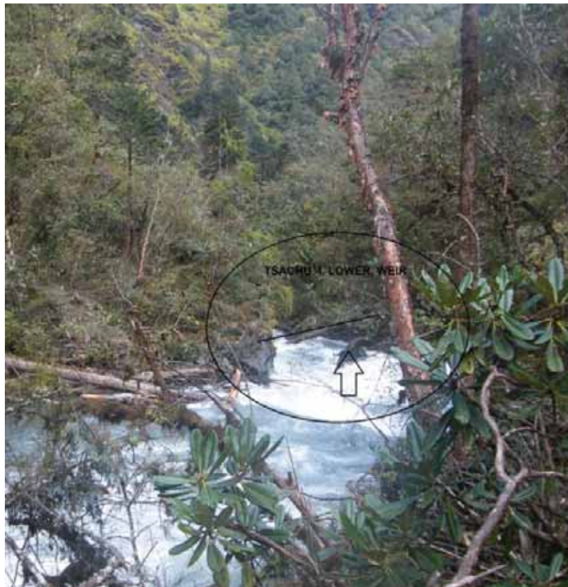
Figure II. 2.4: Barrage site of Tsa chu-I Lower
