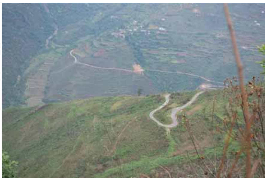
Figure II. 2.21: Powerhouse site of Nyamjang chu
