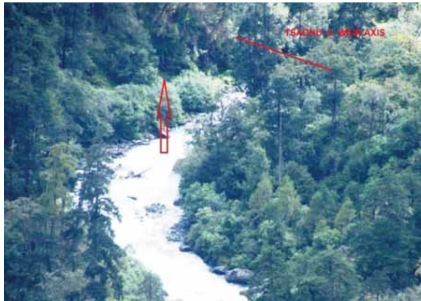
Figure II. 2.6: Barrage site of Tsa chu-II
