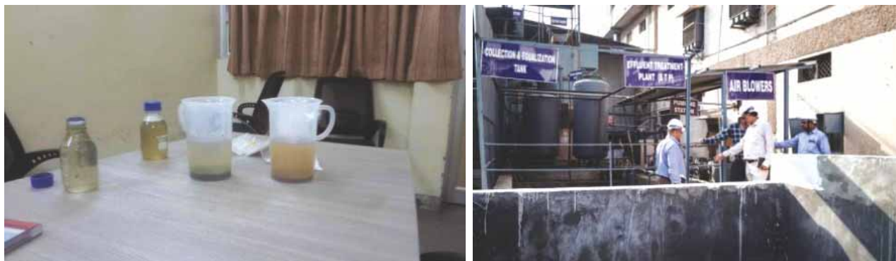
German experts visiting Effluent Treatment Plants
