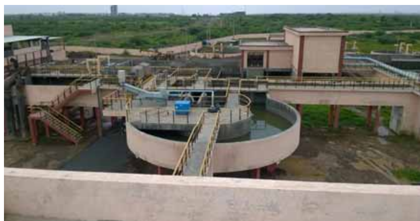
53 mld Sewage Treatment Plant at Gavier, Surat constructed under NRCP
