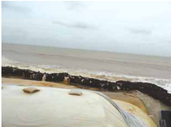
Embarkment of Geo Tubes at Pentha Village
