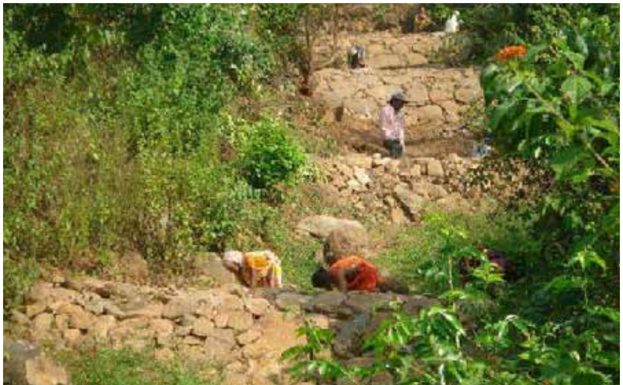
Fig. 4: Checking of land degradation through check dam construction in slope
