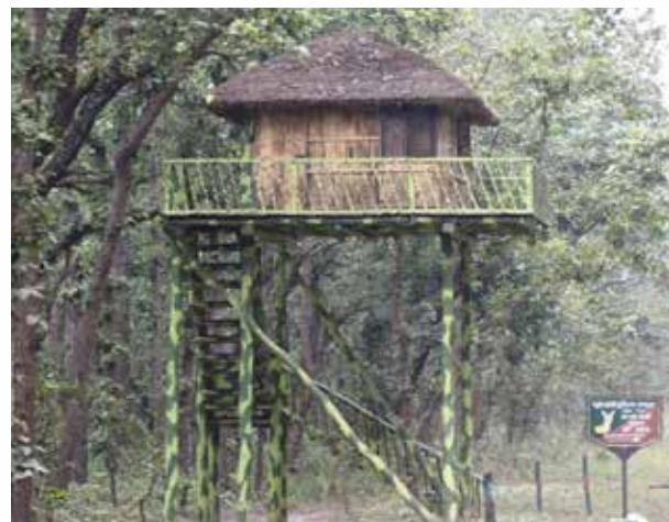
Forest and Wildlife protection works - Watch Towers
