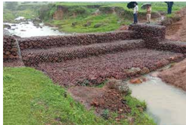
Soil and Moisture Conservation Works 2
