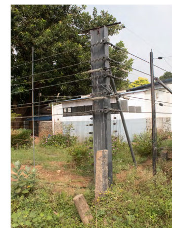
Fig: A steel-rope fence
