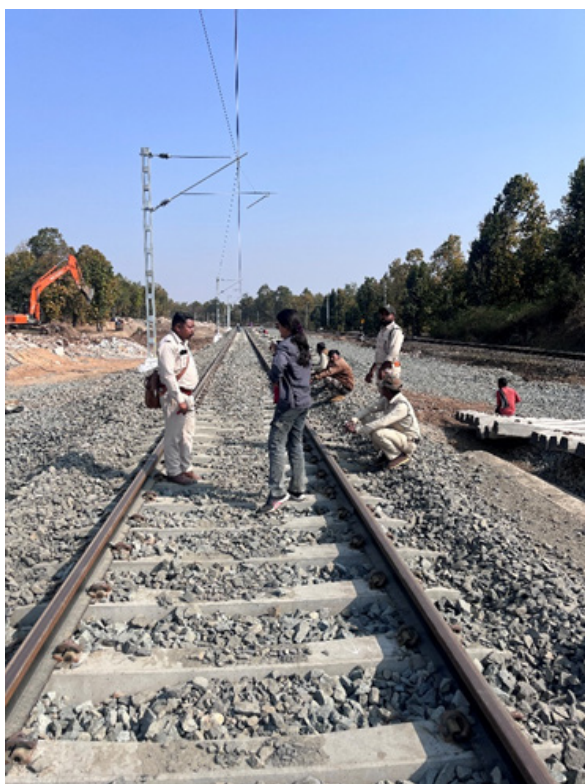
Figure 6: Construction of new railway line on Shahdol Railway segment
