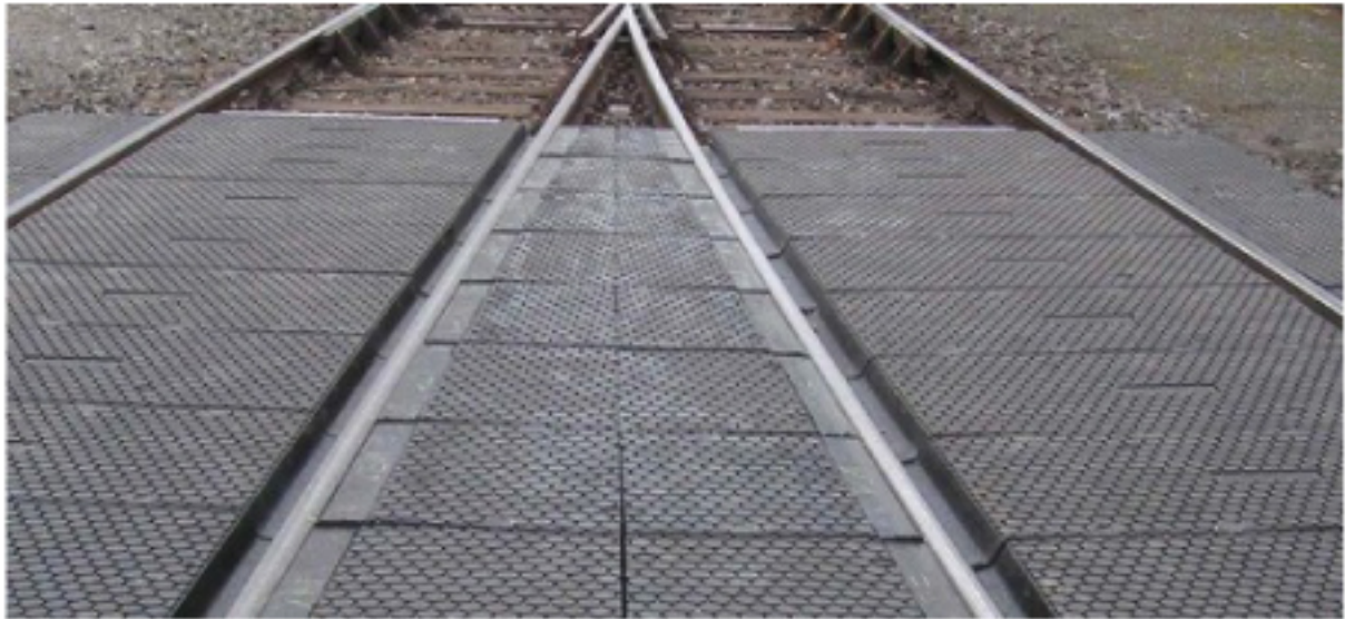
Figure 1. A level crossing with a rubberised surface that can be replicated on level crossings for wildlife.
